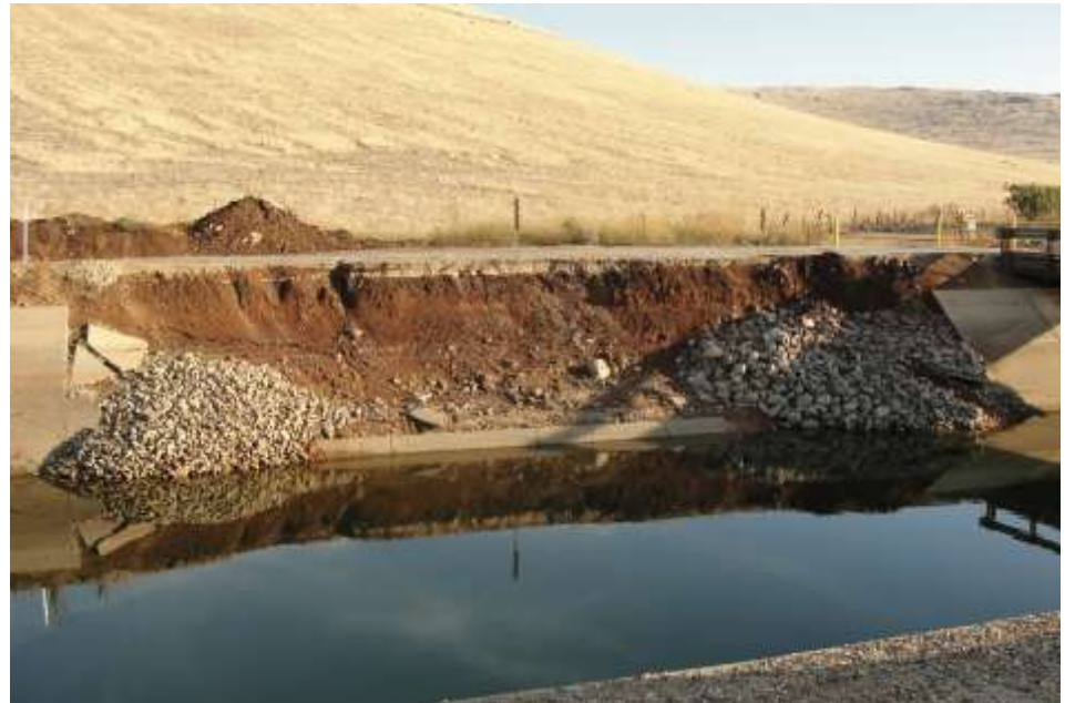
Fig. 2 Typical slide failure, Friant Kern Canal
