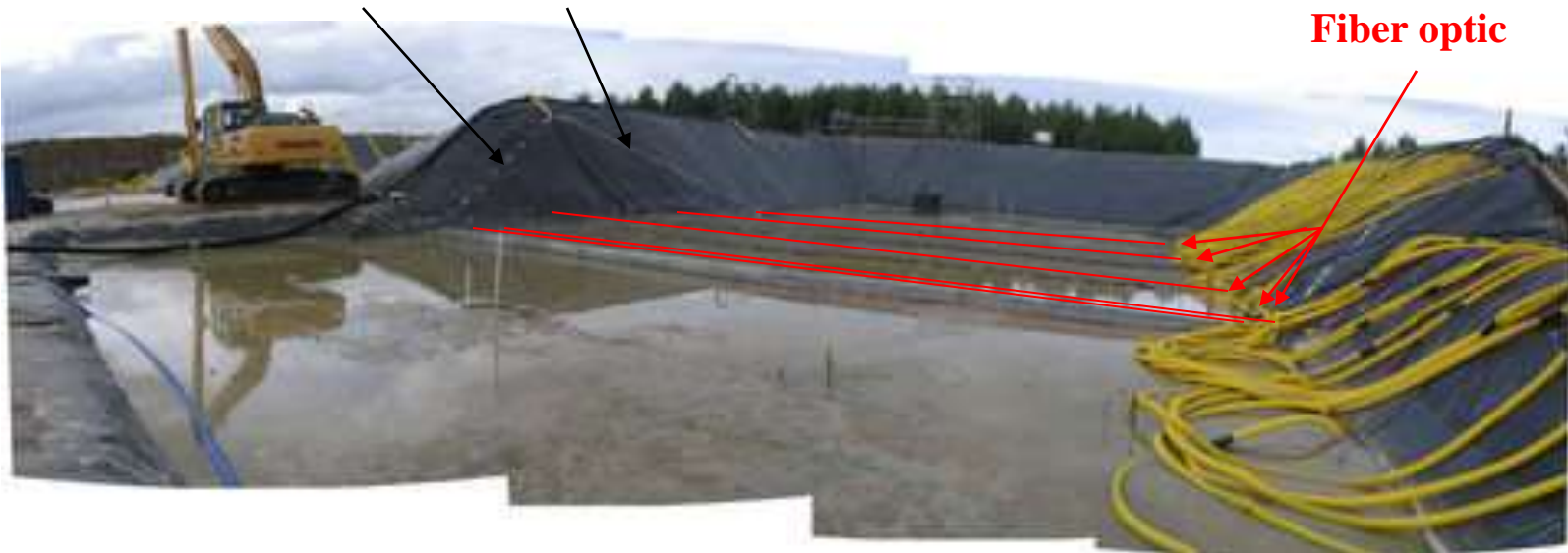
Downstream and upstream of the experimental dam
