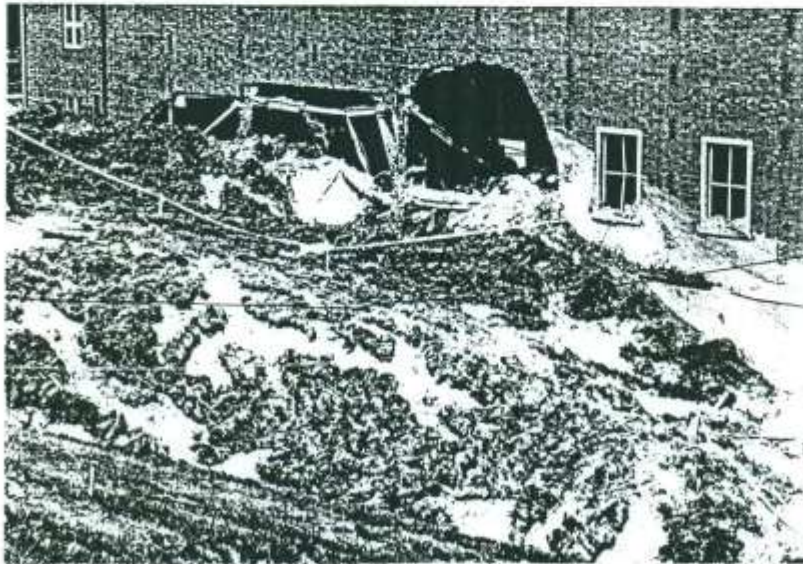
Picture 2. View at the landslide with shifted road and damaged brick wall of the machinery hall
