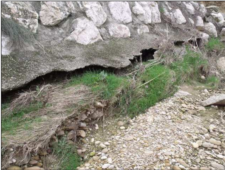
Reach between Garrigues Bridge and the Galet Viaduct (bank protection placed in 2002/3)
