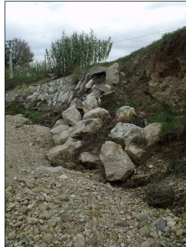
Reach between Garrigues Bridge and the Galet Viaduct (bank protection placed in 2002/3)
