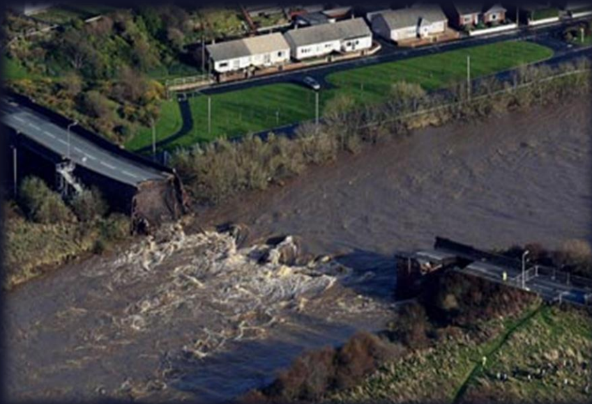
The collapsed Northside bridge in Workington (Cumbria, 2009) ( source: Byrne, 2009 ).
