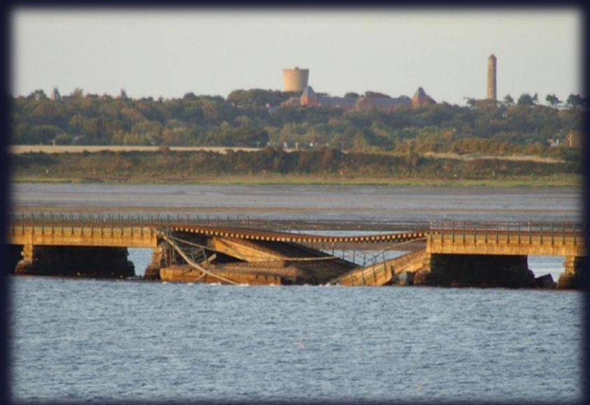
The Malahide viaduct failure (Ireland, 2009) ( source: RAIU, 2011 ).
