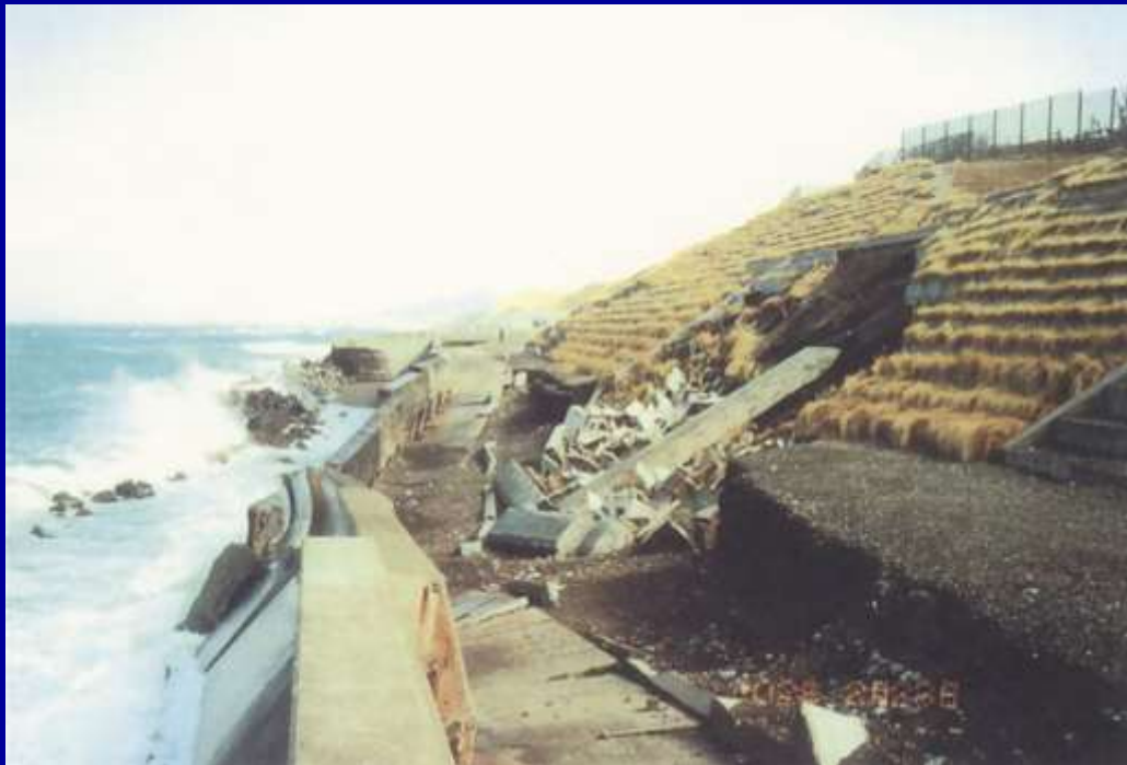
Photo 2: Affected seawall and slope due to severe winter storm (Photograph taken on Apr. 1, 2002: adapted from Hirano (2008)).
