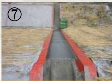
⑦ construct longitudinal ditches
