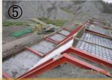
⑤ Construct transverse ditches and RC-platform
