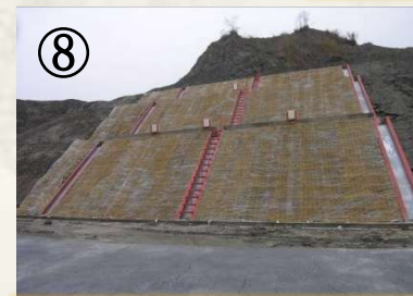
⑧ Put the vegetative mat on the grid and complete the work
