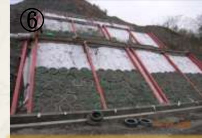
⑥ Place waste tires in the grid and fill with vegetative bags
