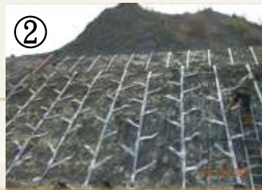
② Install the fabric drain
