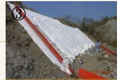
③ Put the geotextile sheet
