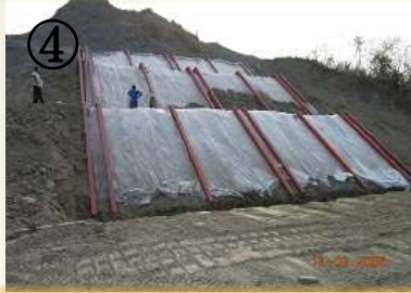
④ Install the grid elements
