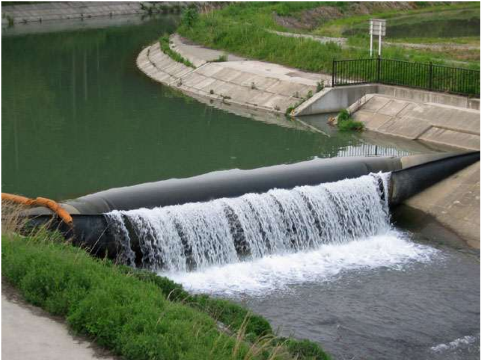
Rubber Dams can function similar to Beaver Dams
