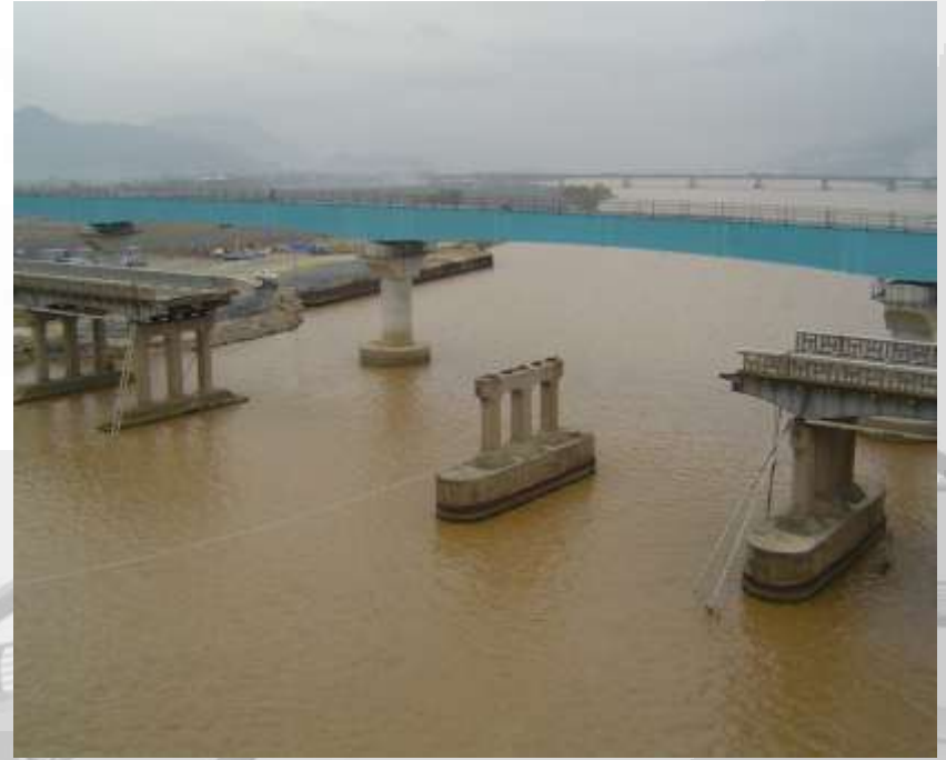
Gu-po bridge failure(2003) Typhoon 'Maemi'
