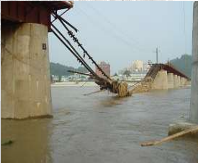
Gam-cheon railroad bridge failure(2002) Typhoon 'Rusa'
