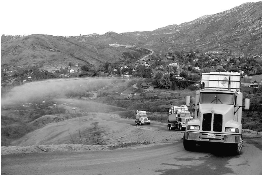
Figure 5. Hydraulic mulch application.
