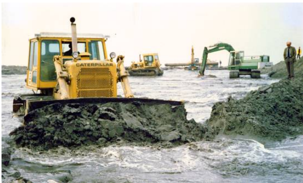
Figure 8 Execution of sand closure
