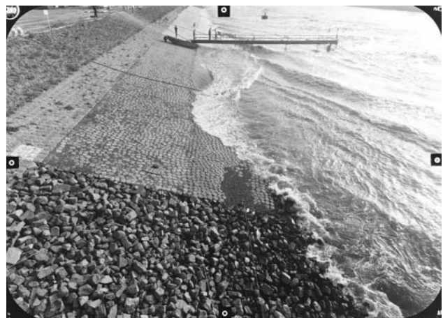
Figure 13. Prototype tests Hartel Canal
