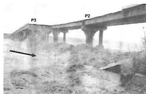
Figure 2(b). Impinging jet downstream of encased pipeline at Houfeng Bridge (Sept. 15, 2008)
