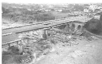
Figure 1. Damage of Houfeng Bridge on Sept. 14, 2008, looking downstream, with flow from right to left
