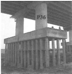
July 2009 (piles exposed around 7.5m)
