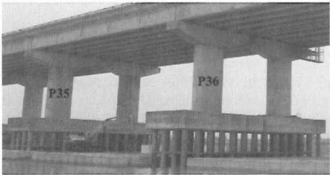
April 2009 (piles exposed around 4.5m)
