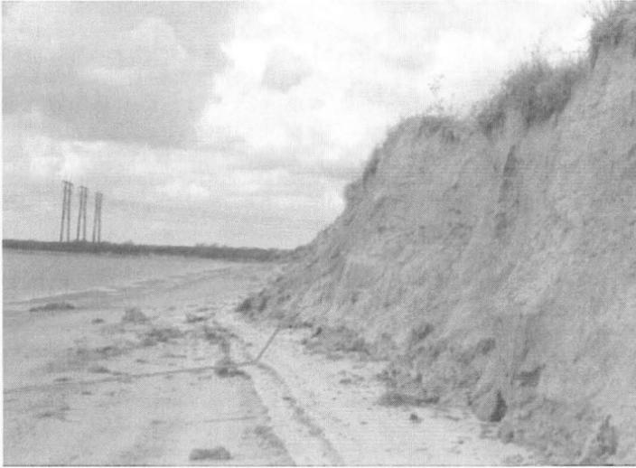
Figure 4. Picture of Phase One embankment after Hurricane Jeanne.
