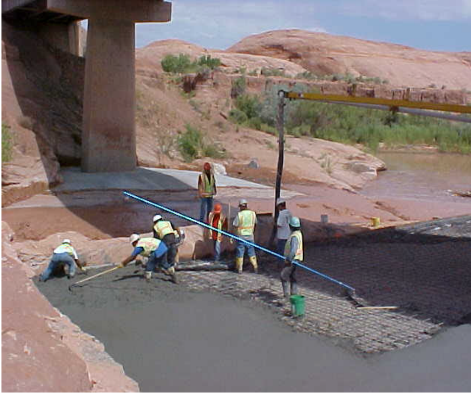
Figure 2 The spread footing foundation after during the installation of the countermeasure
