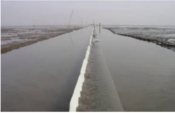
View of pipeline at shore approach during low tide. Note that minor rotation had occurred during pulling operation, partially due to flooding and receding tides. Note scour on both sides of pipeline due to spoiler effects.
