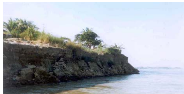
Fig.1 Typical Bank erosion along the Jamuna Right Bank
