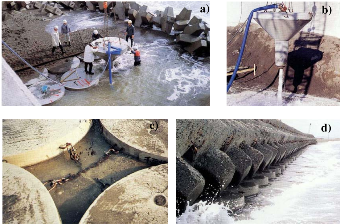
Fig.2. Construction method for top-shaped block foundation
