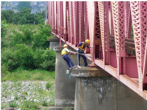
Fig. 8 Setting of the impact vibration test.
