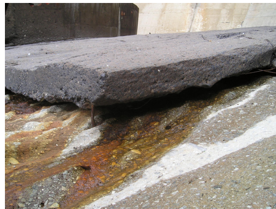
Fig. 2 Photos of damaged concrete apron: a) overview; b) detailed view of damaged concrete slab.
