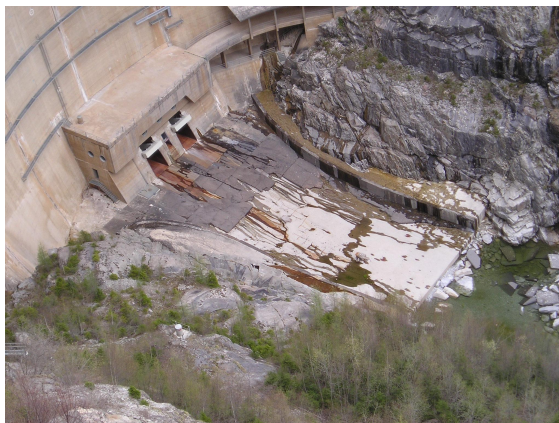
Fig. 2 Photos of damaged concrete apron: a) overview; b) detailed view of damaged concrete slab.
