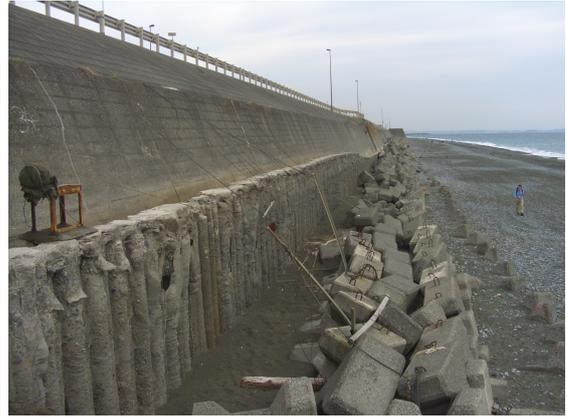
Fig.6 Damaged sea wall at Oiso (Fig.2, #3)
