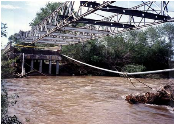
Figure 7: Looking downstream at Bailey Bridge Launching in March, 1995 (photo by Steve Ng, Caltrans)
