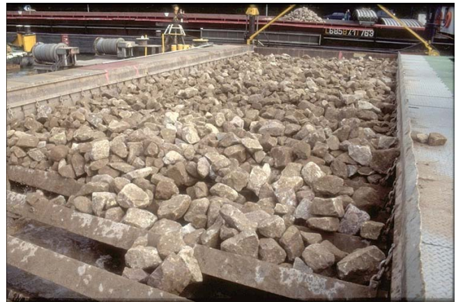
Fig. 10 Stone dumping pontoon
