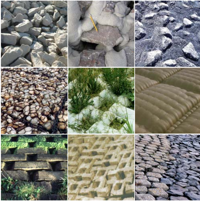
Fig. 7 Armour layers (top left to bottom right: riprap, partial grouted riprap, bitumen grouted riprap, stone mattress, grid concrete mattress, concrete cushion mattress, cable connected concrete blocks, articulated concrete blocks, paved concrete/basalt columns)
