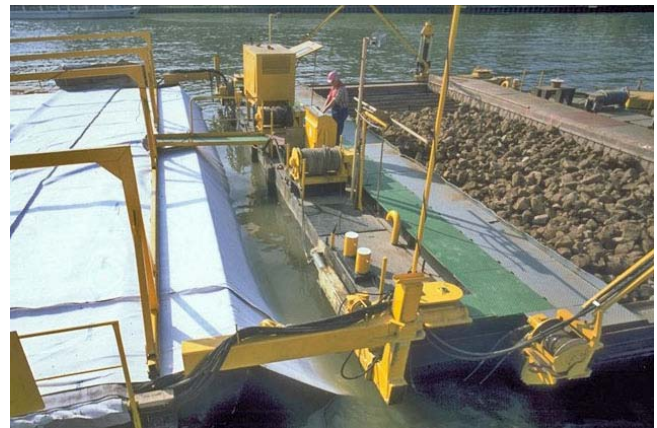
Fig. 11 Geotextile filter placement under water
