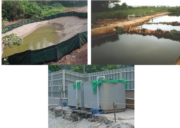
*Sediment basins are an excellent way to trap large volumes of sediment. Unlike silt fence, basins can be designed to handle a large drainage.*
