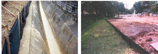
*A silt fence is used to slow down water so it can filter out the sediments carried in the water. They are not intended for a large drainage however and can become overwhelmed. Proper installation and maintenance is essential if it is to be effective.*
