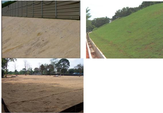
*Temporary covers /seedings during construction or while individual lots wait for new stages is an excellent way to control soil erosion.*
