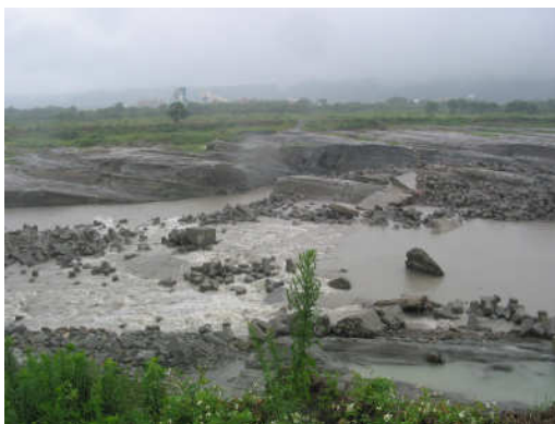
Figure 1(c). Eroded tetrapods downstream of bridge
