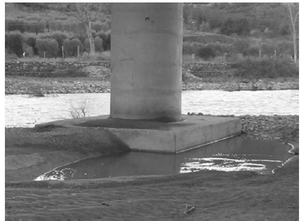
Figure 1. River Basento (Italy): Local scour around the plinth of a pier founded on piles
