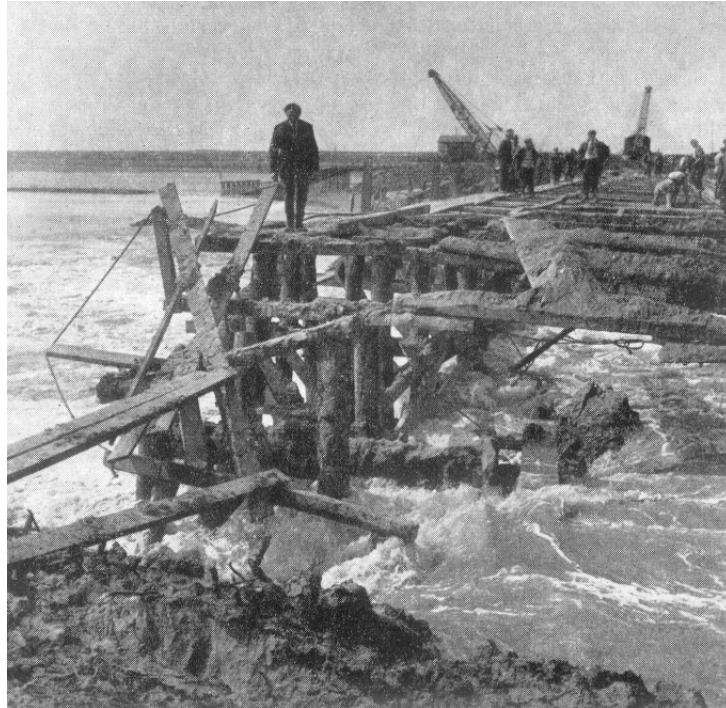
Figure 3. Breach of the clay-filled cofferdam at the east abutment a few minutes prior to High Water [4].
