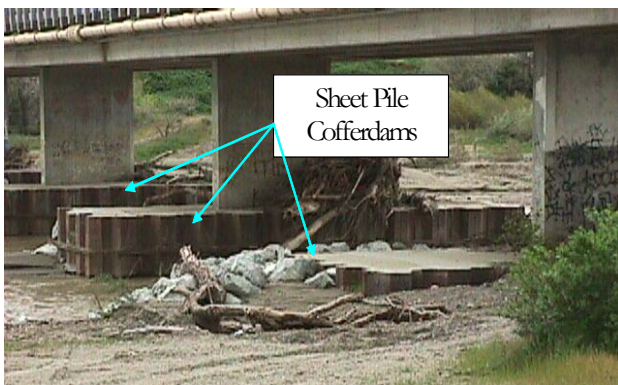
Figure 14: Cienega Road Bridge looking upstream at the sheet pile cofferdams (photo by Author)
