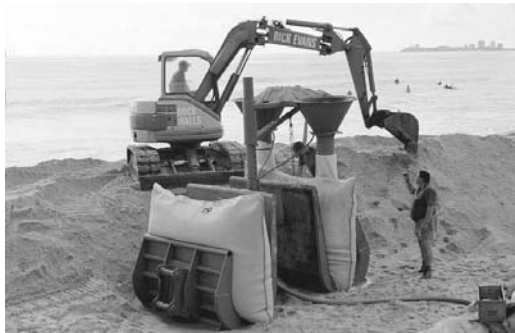
Figure 8. Filling and transport of 2,5m 3 containers in special buckets (Geofilters Australia)
