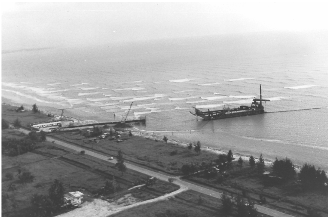
Fig 2. Dredging of the pipe trench with cutter suction dredging in progress; on shore is the pipeline landfall; in the foreground is the Pan Sarawak Coastal Highway, behind the dredger is the wave interference pattern with breaking waves.
