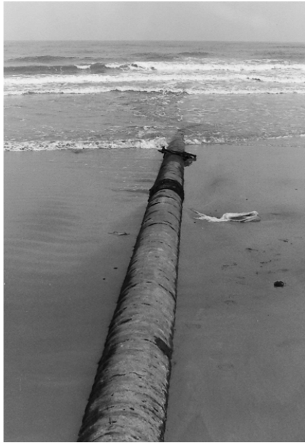
Fig 7. Exposed pipeline
