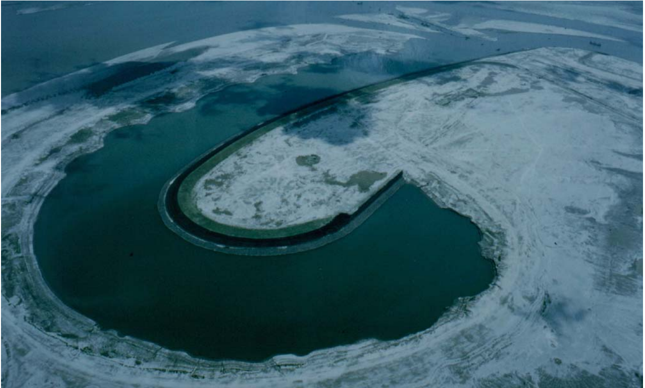
Figure 19. The western, 3.2 km long, guide bund, seen from the North (upstream) after its completion (April 1997). The 5 km long bridge is still under construction in the background. The picture is dominated by the wide, 27 m deep, trench, especially dredged to enable construction of the gentle (1V:5H to 1V:6H) under water rip rap slope. Above water on the slope one can see, intersected by a narrow berm, the black strip of the open stone asphalt and the hand-placed riprap
