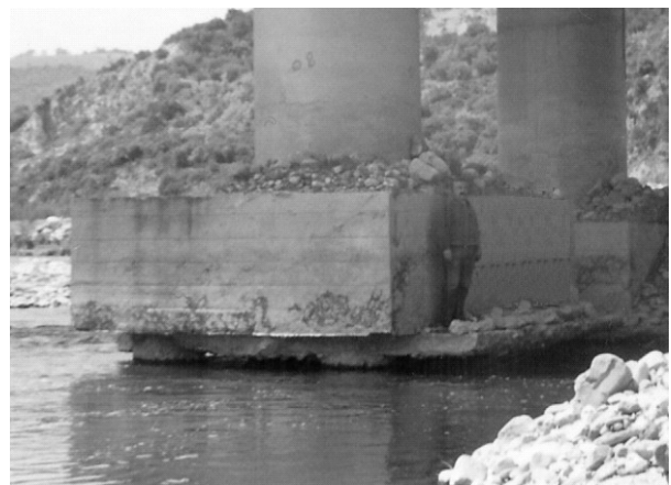
Figure 2. River Basento (Italy): General scour around a pier with consequent exposure of the piles
