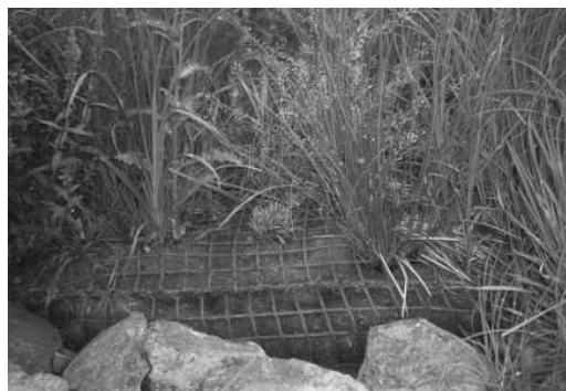
Figure 4. Pre-planted rope gabions
