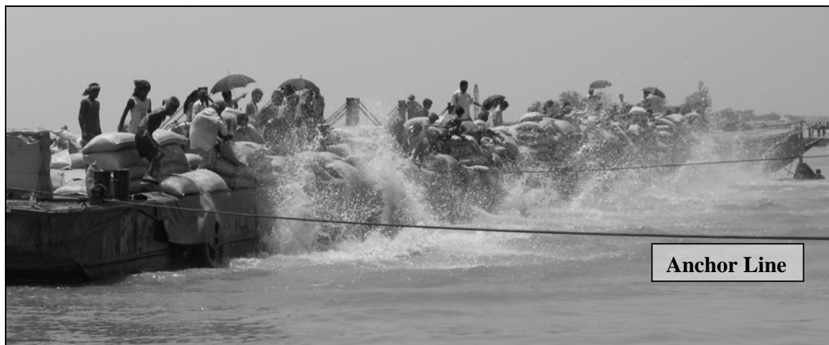
FIGURE 7 1 ST LEVEL PROTECTION DUMPED FROM POSITIONED BARGES
