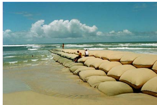
Figure 9. Sea groyne of geotextile containers (Hornsey)
