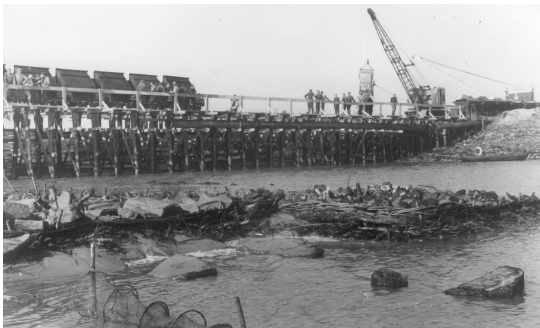
Figure 2. The tidal closure, effected by means of a cofferdam filled up with clay during the rising tide
