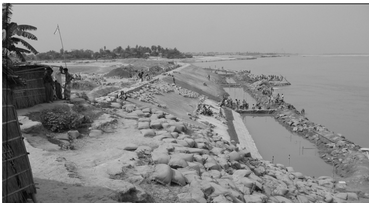
FIGURE 8 CONSTRUCTION OF PERMANENT WAVE PROTECTION ABOVE LOW WATER LEVEL DURING THE ADAPTATION PHASE
