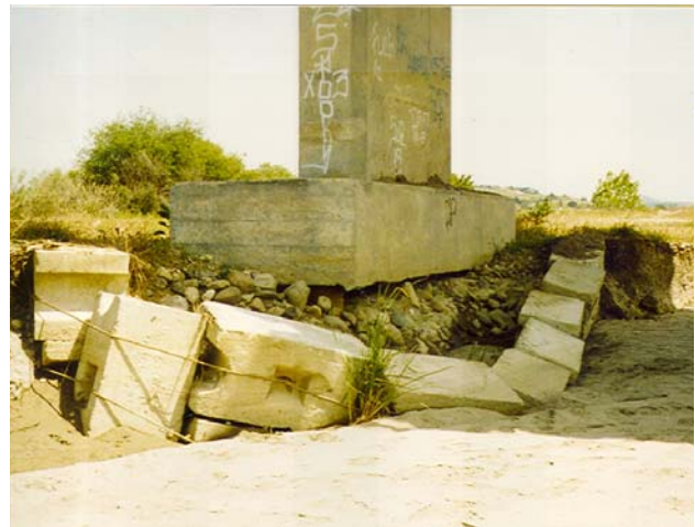
Figure 11: Pier #5 undermining and failure of “scour protection” installed in 1989 (photograph by Caltrans)
