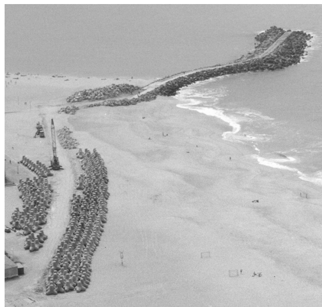
Figure 7. Reconstruction of the North groin of Espinho, 1997.
