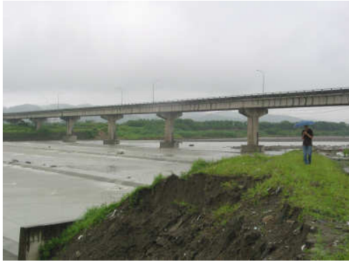
Figure 1(a). Concrete apron as a pier-scour countermeasure at a bridge in Taichung, Taiwan
