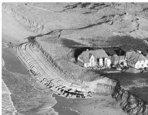
Figure 3. Wrapped wall protection of the Sylt coastline (Naue)
