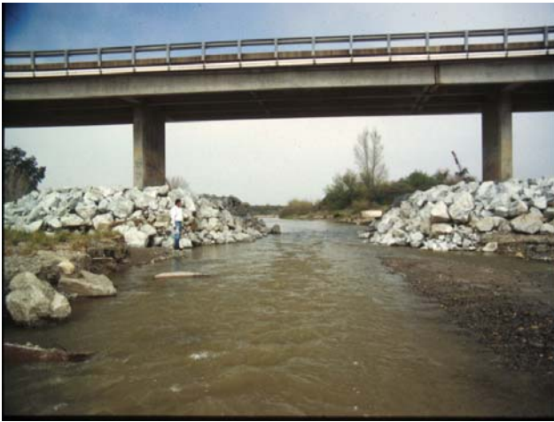
Figure 13. Cofferdams and rock rip rap placed following 1995 Storms (photo by Mussetter Engineering, Inc.)
