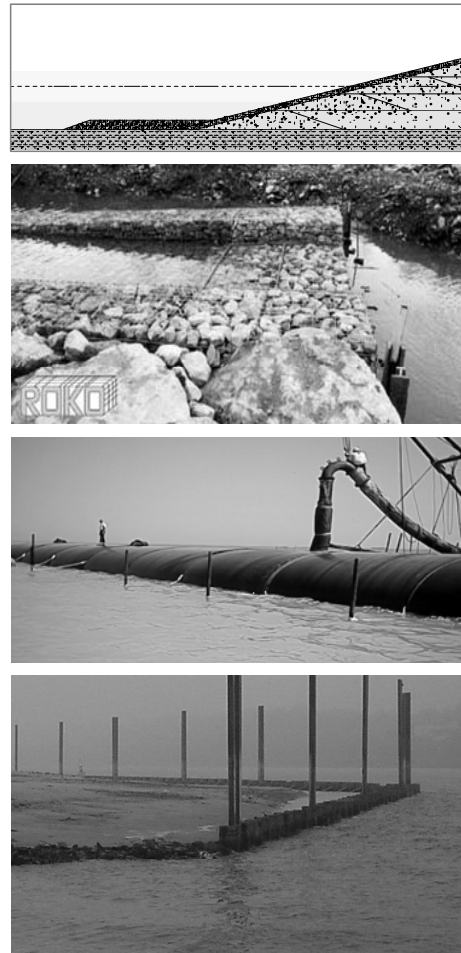
Figure 4: Construction types for the bordering dam
