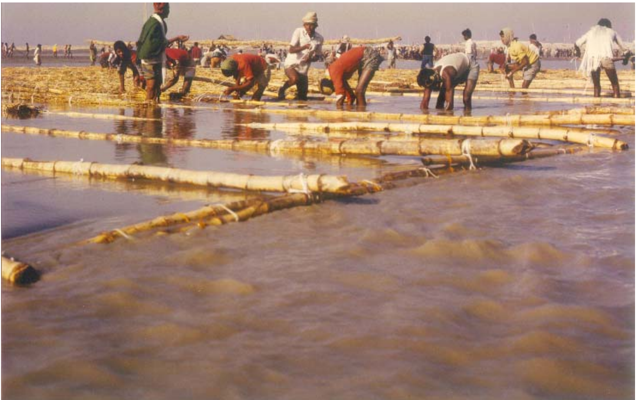
Figure 13. Making a bed protection mattress on the shoals at low tide
