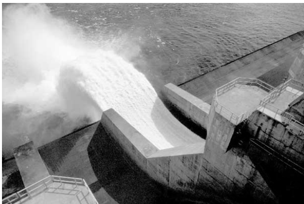
Figure 1. a) Detailed view of flip bucket spillway; b) General view of spillway and plunge pool
