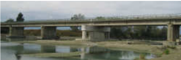
Figure 4 The bridge after retrofitting of pier P2 (Downstream view)
