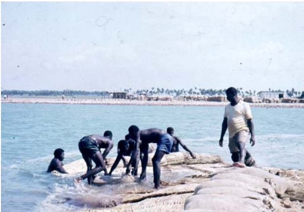
Figure 8. Slope protection at end of dam
