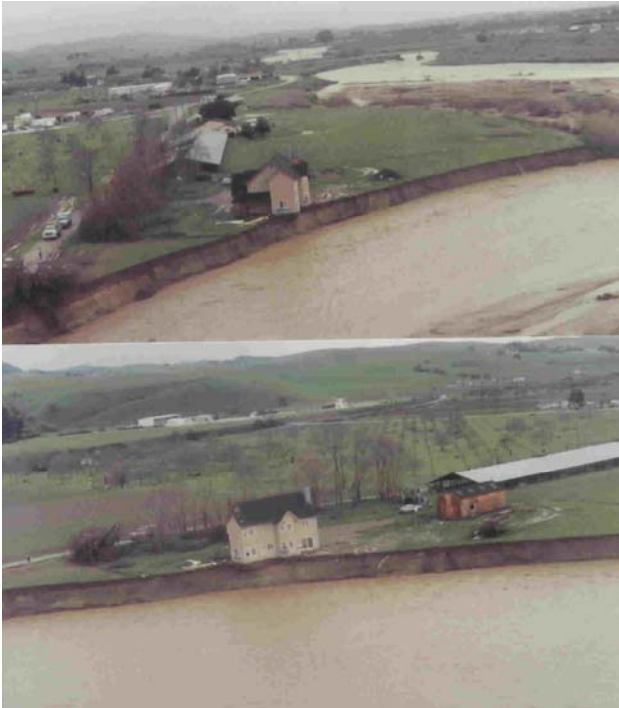
Figure 9: Lateral channel erosion undermined the foundations of a house on the San Benito River (photo by San Benito County Public Works Department)
