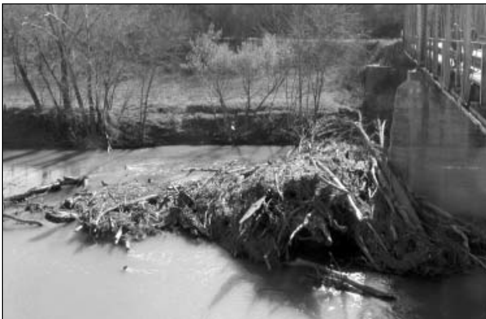
Figure 4. Debris pile with conical profile geometry.
