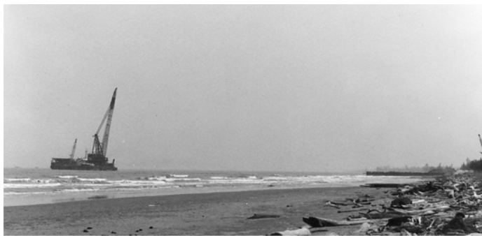
Fig 4. LB 26 pulling pipe to shore
