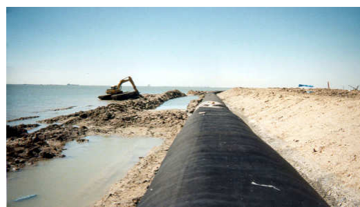
Figure 2. Geotextile tube for coastal scour protection (to be covered by sand) (Bradley)
