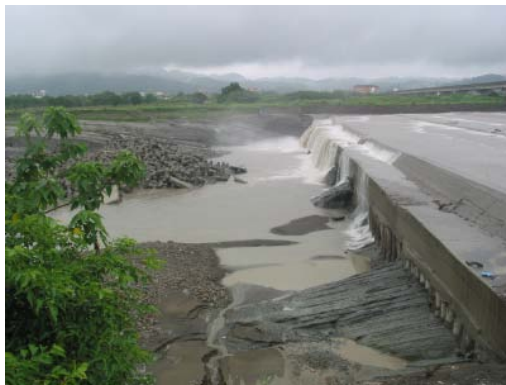
Figure 1(b). Edge failure leading to erosion of the tetrapods
