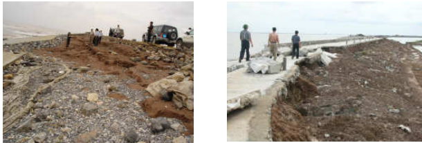
a. damage of armour layer and erosion upper part of outer slope
